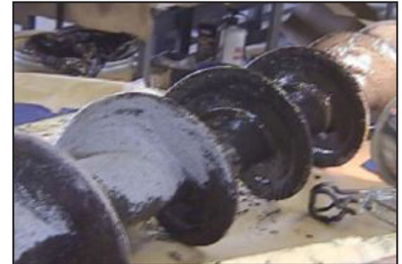
Completed screw coated with ARC BX1* and topcoat with ARC 855
